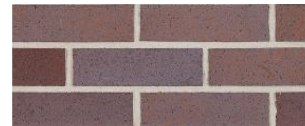
First Floor + Recesses Deep Brick
