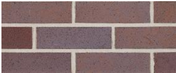
First Floor + Recesses Deep Brick
